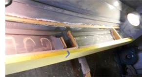
There are several ways to fasten the tanks. Since the epoxy will seal and hold, nails screws or staples are just clamps. You can use 5/8" or 3/4" boat nails with 3" spacing and leave them in the boat. Another way is to use 1/4" crown staples (steel is OK) with a 4mm to 1/4" tack strip. After the epoxy has set the staples are removed, leaving only small holes to putty. The same can be done with #6 screws with 1/4" plywood pads under the screw head.
