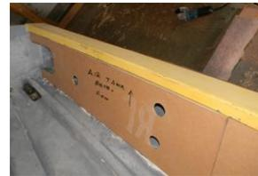
Seal the back side of the tank walls with epoxy.
